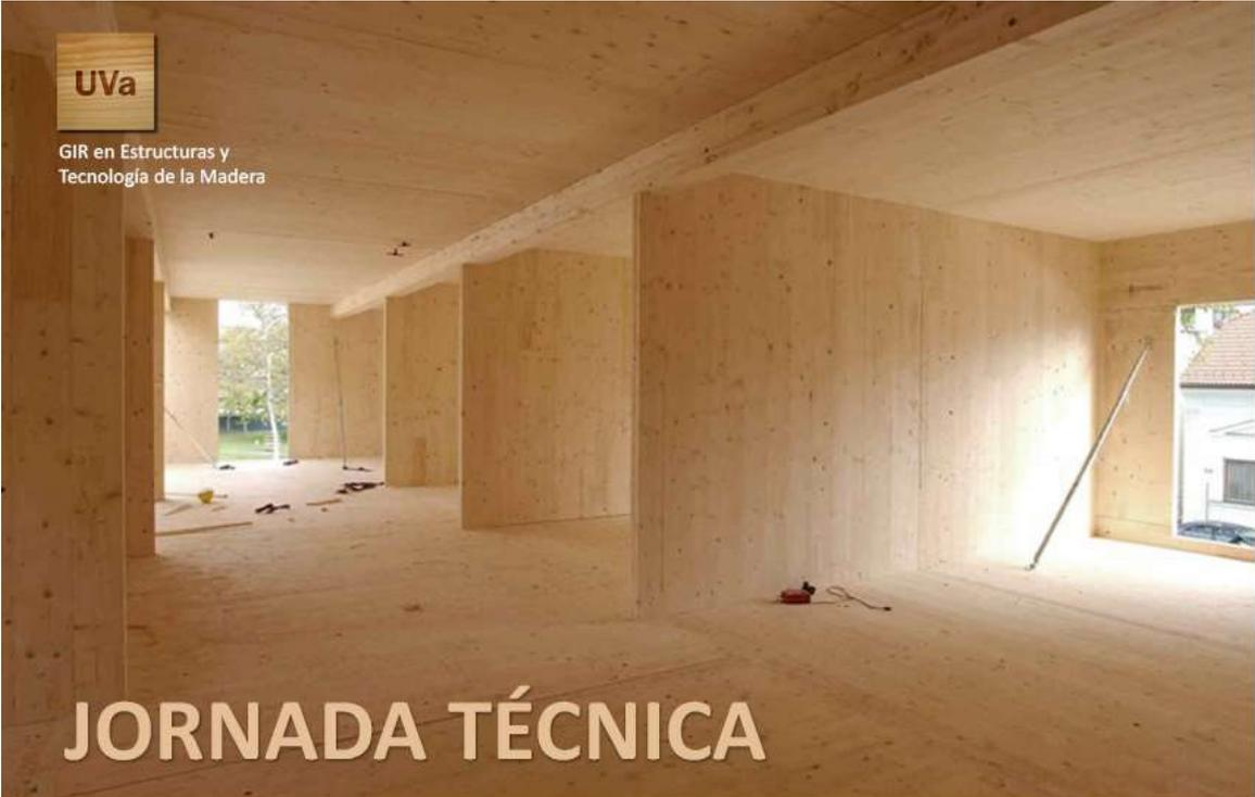
A photograph showing the interior of a building under construction. The walls, ceiling, and floor are made of light-colored wood panels (CLT). The space is open, with several large windows and doors. A long metal pole leans against the wall on the right. The lighting is warm and natural, coming from the windows.
